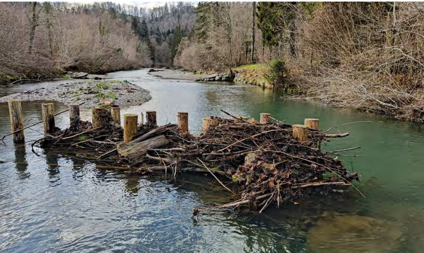
Fig.11: Engineered logjam at the Töss River, Switzerland.
