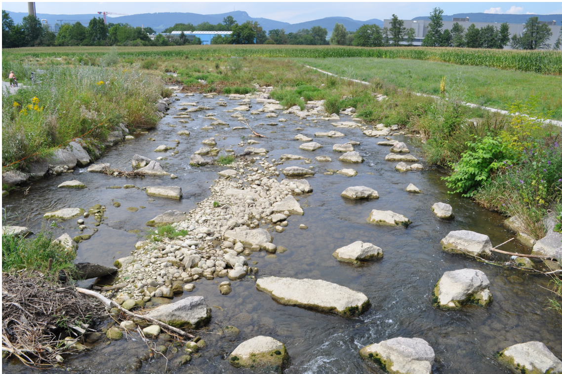
Figure 6.3 UBR at the Wyna River with a specific discharge of q \approx 0.03 \text{ m}^3/(\text{s m}) corresponding to one of the smallest discharges measured in 2012, approximately corresponding to Q_{30} (view in flow direction).
