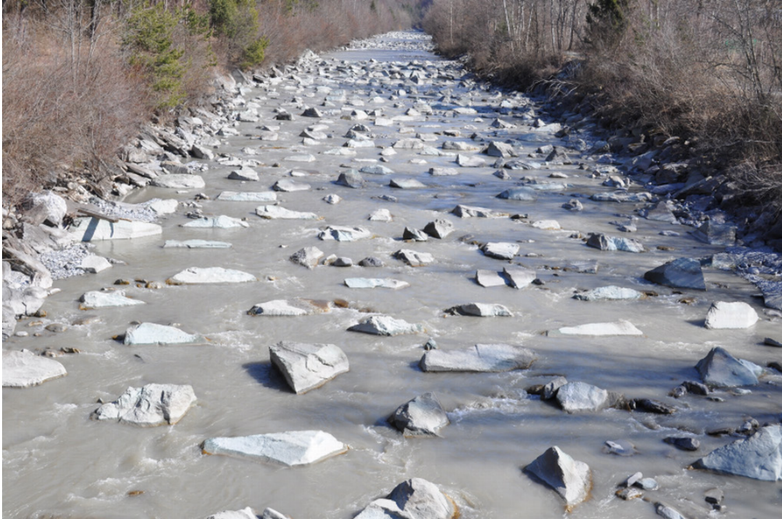
Figure 1.1 Unstructured block ramp at the Landquart River with specific discharge q \approx 0.28 \text{ m}^3/(\text{s m}) , corresponding approximately to Q_{30} (view against the flow direction).
