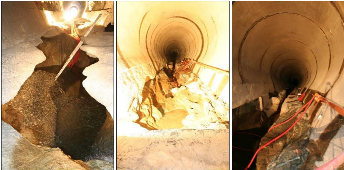
Figure 2: Eroded invert concrete and underlying Gneiss rock (2011)
