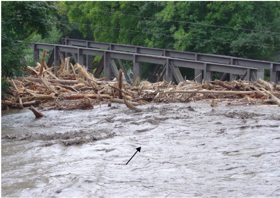
Figure 2.8 2005 flood in Switzerland, LW accumulation at a bridge in Canton Obwalden (Photo: belop GmbH)
