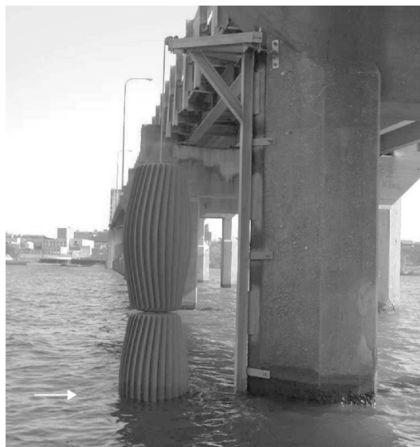
Figure 3.13 Double-stacked installation of a LW sweeper at the Mississippi River, USA (adapted from Bradley et al. 2005)
