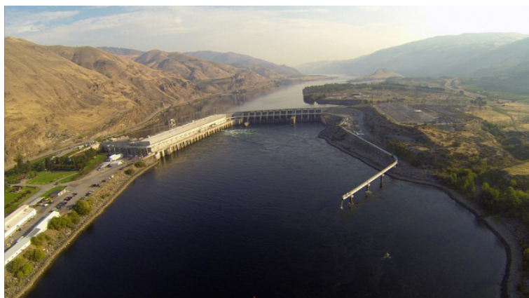
Figure 2.15 Rocky Reach Dam with bypass tailrace outlet at Columbia River, Washington (Photo by Chelan County PUD), view against flow direction
