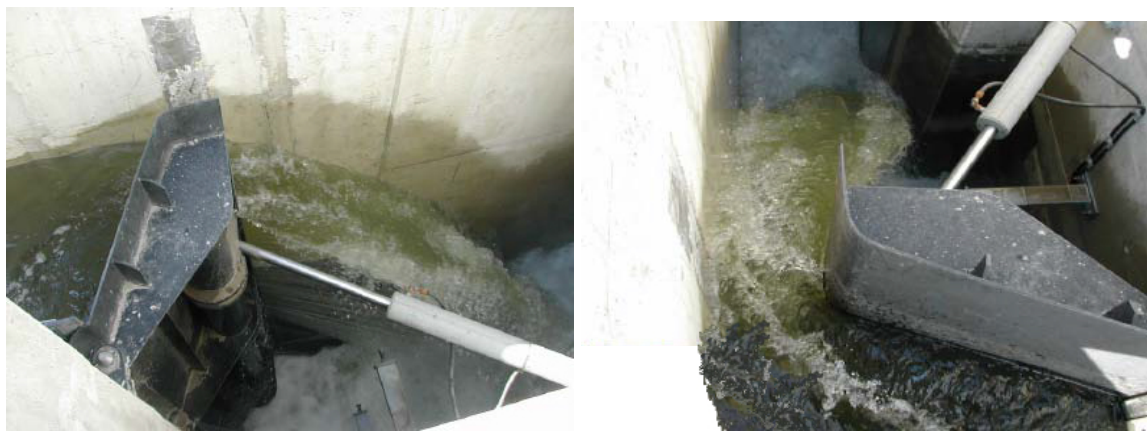
Figure 2.14 Vertical axis flap gate at the bypass entrance with a top and a bottom opening constructed with gradual geometric transitions to achieve a gradual velocity increase, adapted from BAFU (2012)
