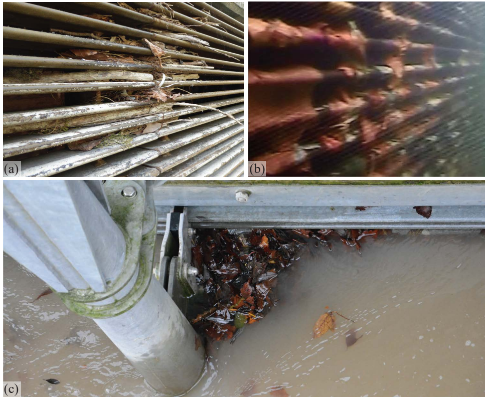
Fig. 9.1: (a) Permanent clogging at the vertical tie-bars of the residual flow HPP Schiffmühle during drawdown in July 2018 (Photo: J. Meister), (b) underwater picture of foliage clogging at HPP Stroppel in October 2016 (adapted from Zaugg and Mendez, 2018), and (c) operation of RCM at HPP Hard during a flood event on 03.12.2018 (cleaning direction from left to right; Photo: J. Meister); the clear bar spacing of all three HBRs is s_b = 20 mm
