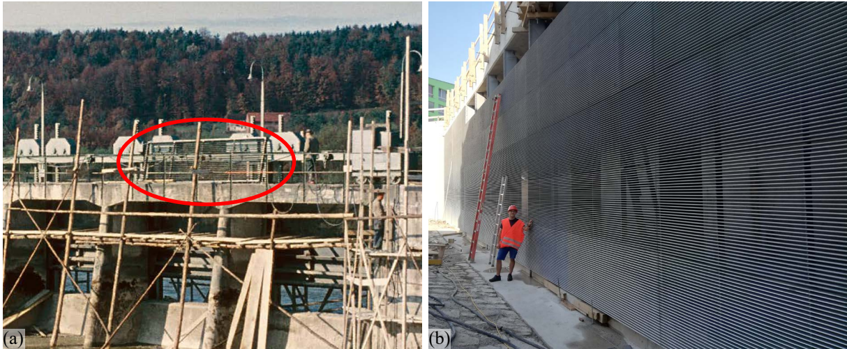
Fig. 3.1: (a) Construction of Hirten weir and an HBR field (encircled in red) in 1922 (courtesy of Wacker Chemie AG) and (b) HBR at the main HPP Dietikon in July 2019, shortly before it started its operation (Photo: H. Fuchs)
