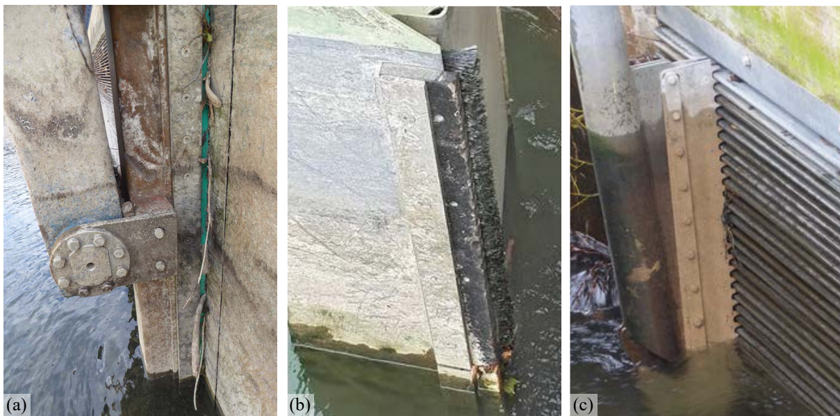
Fig. 3.8: RCMs of HBRs with (a) a plastic scraper (residual flow HPP Schiffmühle), (b) a brush (residual flow HPP Rühlig, 47°23'56.4"N, 8°03'07.3"E), and (c) a rake (HPP Hard) (Photos: J. Meister; adapted from Meister et al. , 2018a)
