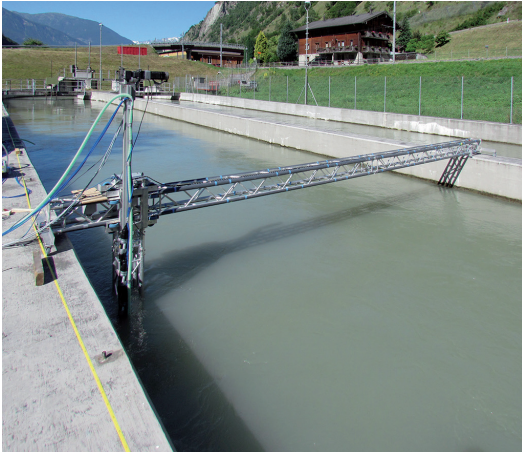
Measuring campaign at Mörel sand trap at KW Massaboden SBB (Photo: C. Paschmann, VAW)
