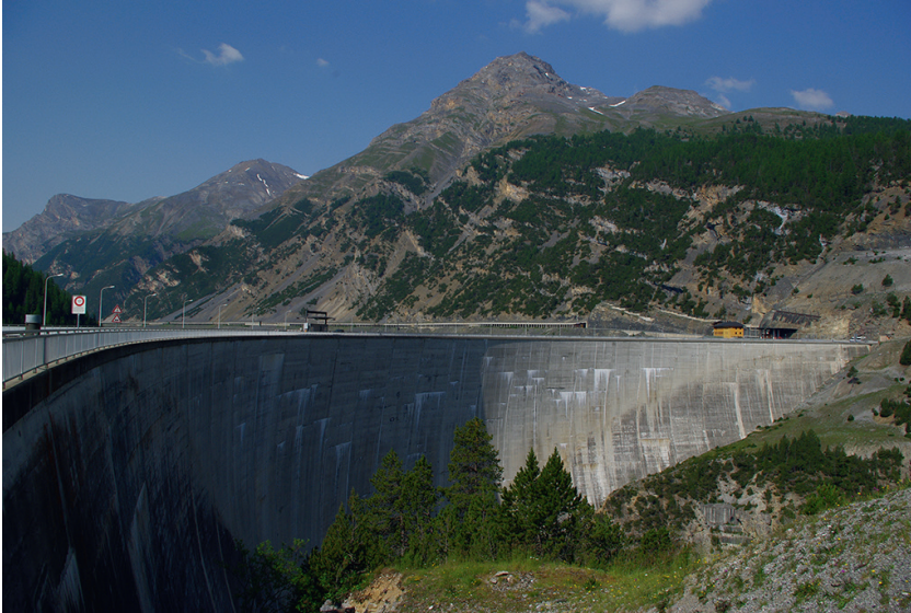
Punt dal Gal dam in Switzerland (Photo: M. Bühlmann, VAW)
