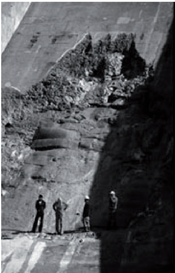
Fig. 1: Cavitation damage on Karun dam, Iran
