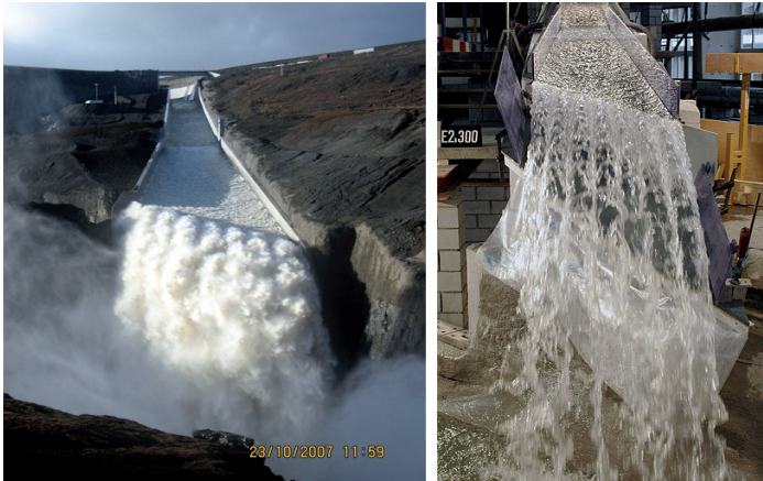
Fig. 1: Spillway chute with jet for 300 m 3 /s in the prototype (picture: Landsvirkjun) and in the model.
