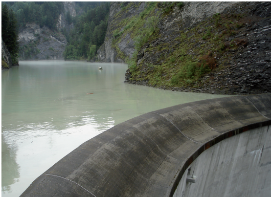
Dam crest of the 61 m high Solis Dam with the reservoir
