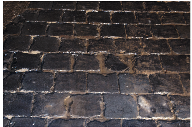
Abraded cast basalt tiles in the Pfaffensprung SBT (M. Müller-Hagmann)
