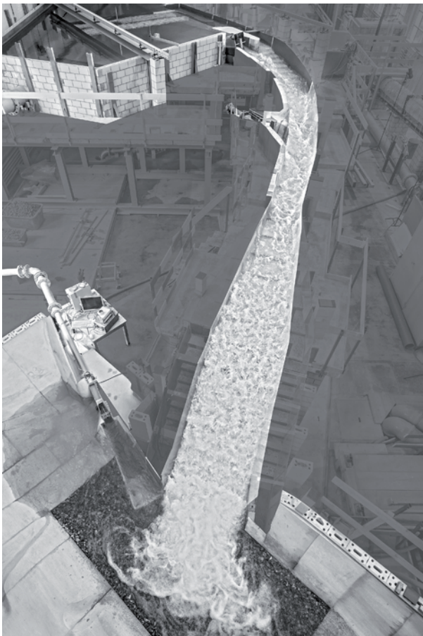
General flow conditions on the stepped spillway for the design flood.
