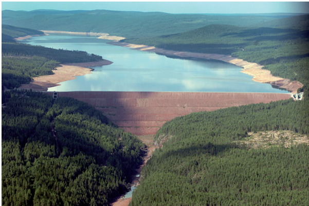
Trängslet dam with the existing spillway located at the left abutment (Picture: Fortum Power AB).
