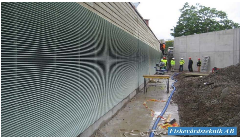
Fig. 1: FGS with horizontal bars at Herting Hydropower Plant, Norway (Photo: Olle Calles)
