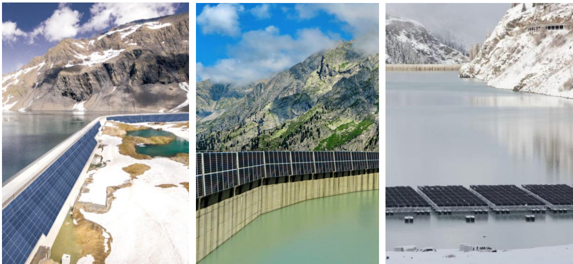
Fig. 1: Renderings of PV installed at Muttsee dam, 2474 m a.s.l. (Axpo Power AG), and Albigna dam, 2165 m a.s.l. (EWZ), floating PV test rig on Lac des Toules, 1810 m a.s.l. (Romande Energie)
