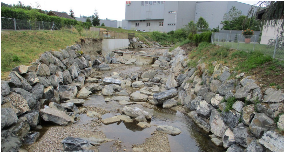
Fig. 1: Remnants of the block ramp after its failure during a flood event in May 2023.
