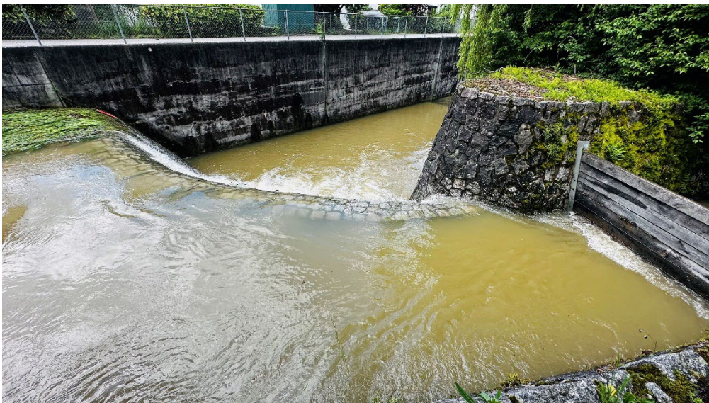
Fig. 1: Eulach river, intake of the flood retention tunnel (Source: AWEL)
