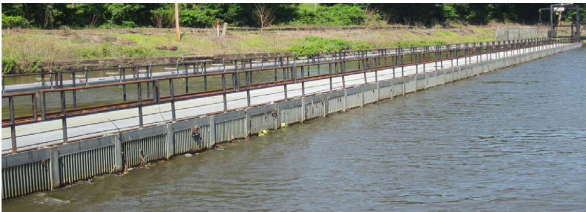
Fig. 1: Example of a 'fish-friendly' guidance screens (FGS), Holyoke Canal, Connecticut River, USA (Source: VAW)
