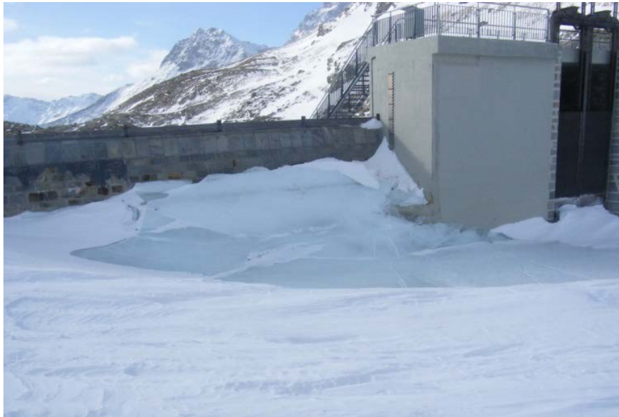
Fig. 1: Ice pressed against the Lago Bianco dam (Source: BFE)
