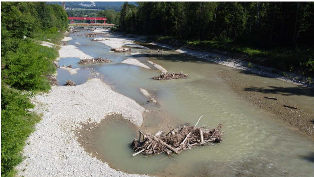
Fig. 1: Engineered logjams at the Emme River close to Solothurn (photo by IUB Engineering).
