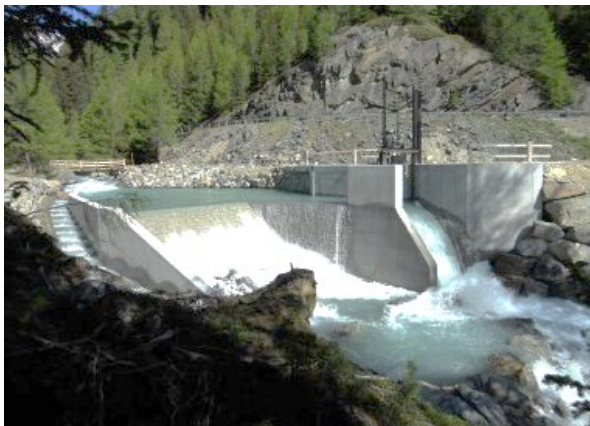
Fig. 1: Intake of HPP Susasca (Source: Hydro-Solar Water Engineering AG)
