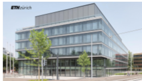
BSS Building - Home of the D-BSSE since 2023
