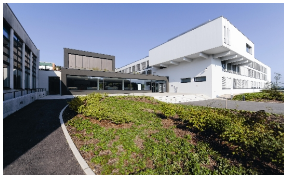
Figure 1: The conference center: Campus Sursee, Switzerland.
