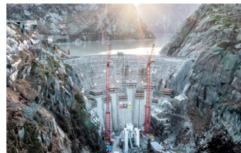
Spittallamm Dam, © David Birri
