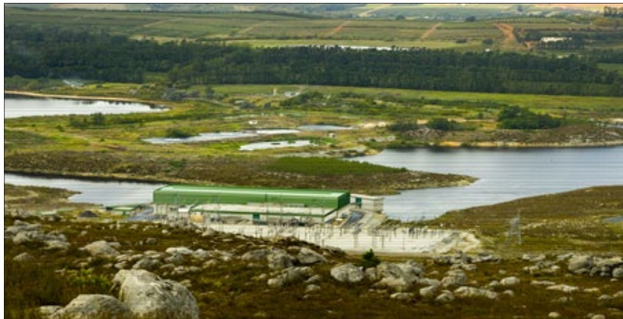
Images: Eskom website http://www.eskom.co.za/AboutElectricity/VisitorCentres/Pages/Palmiet_Pumped_Storage_Scheme.aspx
