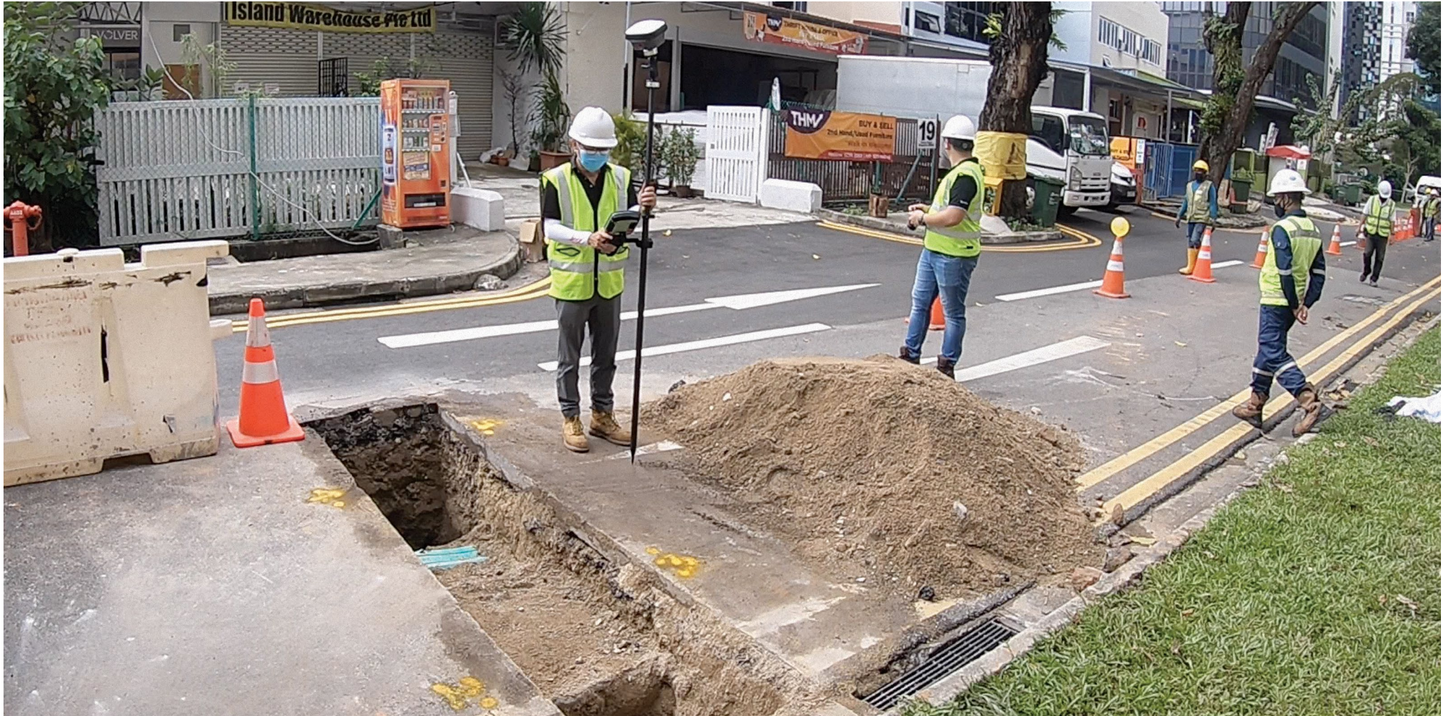
Image-based measurement of exposed utilities using the Leica GS18i
