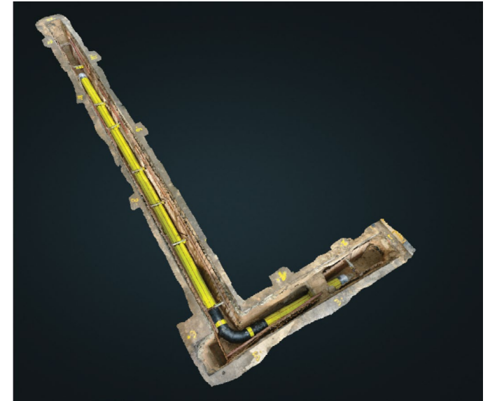
3D mesh model of a newly installed gas pipe
