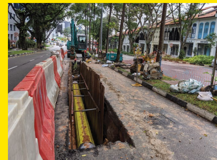
Gas pipe laying works on Cantonment Road.
