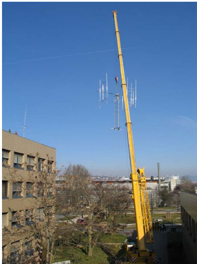
Figure 22: Hoisting the antennas and mast of the EPFL ground station.
