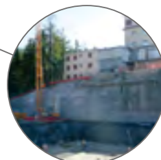
Complex excavation safety – reinforced and prestressed shotcrete wall.
