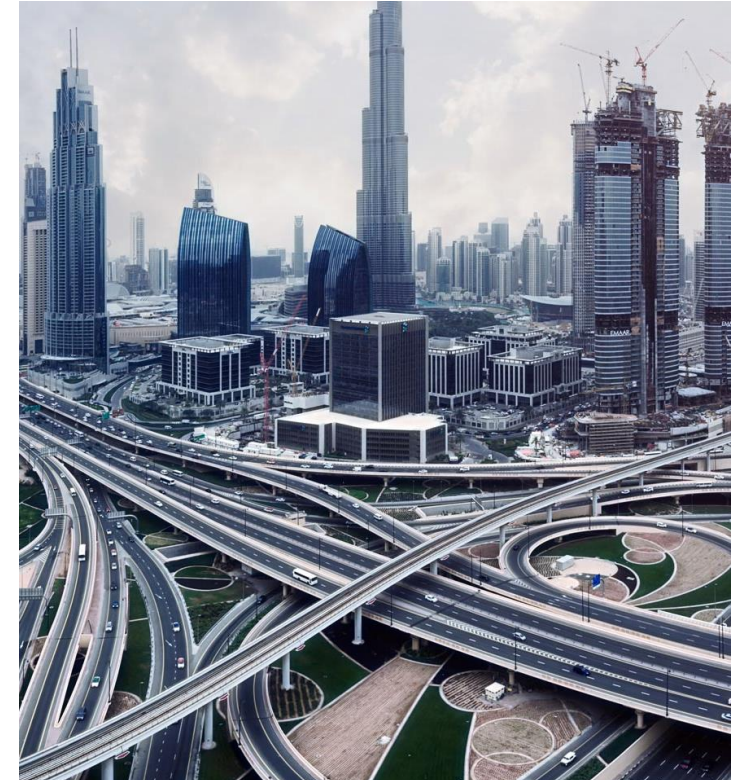
Sheikh Zayed Road, Dubai (Avaya)
