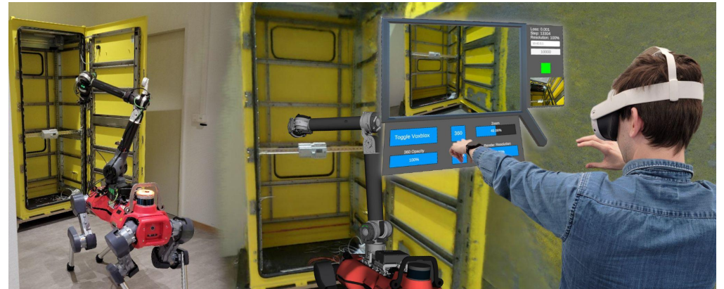
NeRF render of a switchboard cabinet captured on ALMA, being used by a VR teleoperator
