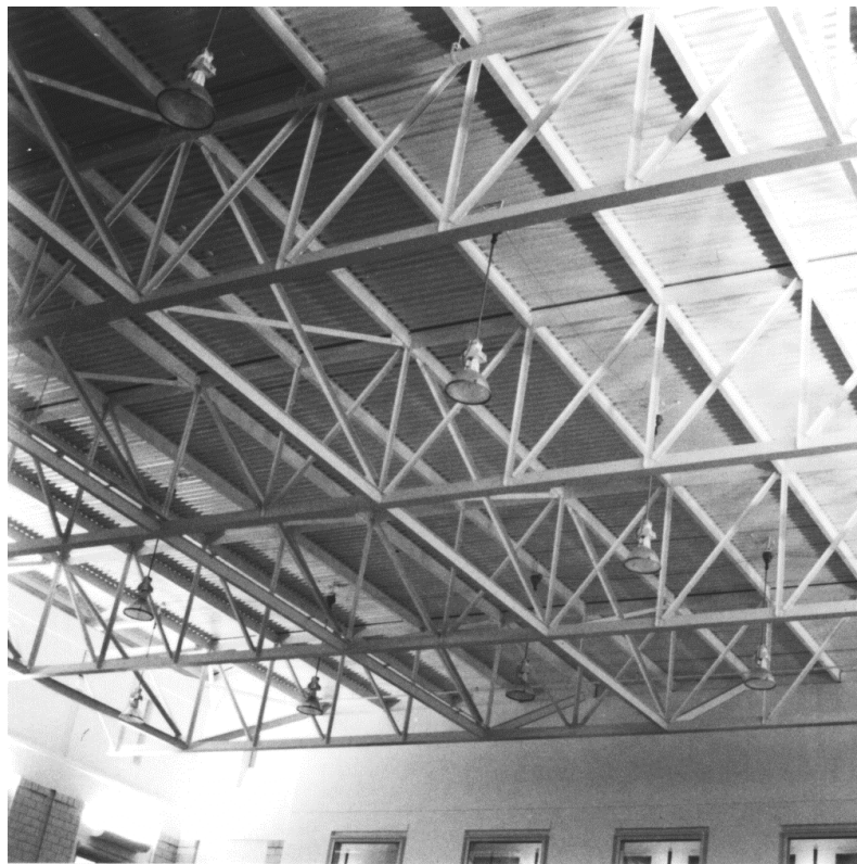
Figure 7.4: Roof truss system
