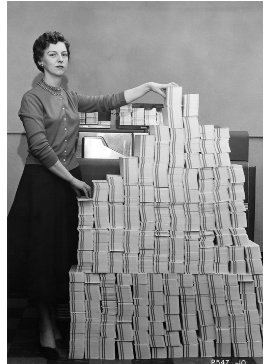
This stack of 62,500 punched cards — 5 MB worth — held the control program for the giant SAGE military computer network. ( link )
