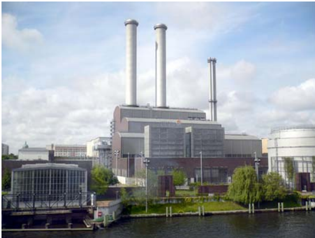
Combined Heat/ Power Plant (CHP), Berlin-Mitte
