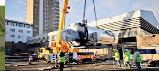
3 High efficient thermal gas boilers (4.9MWh)
