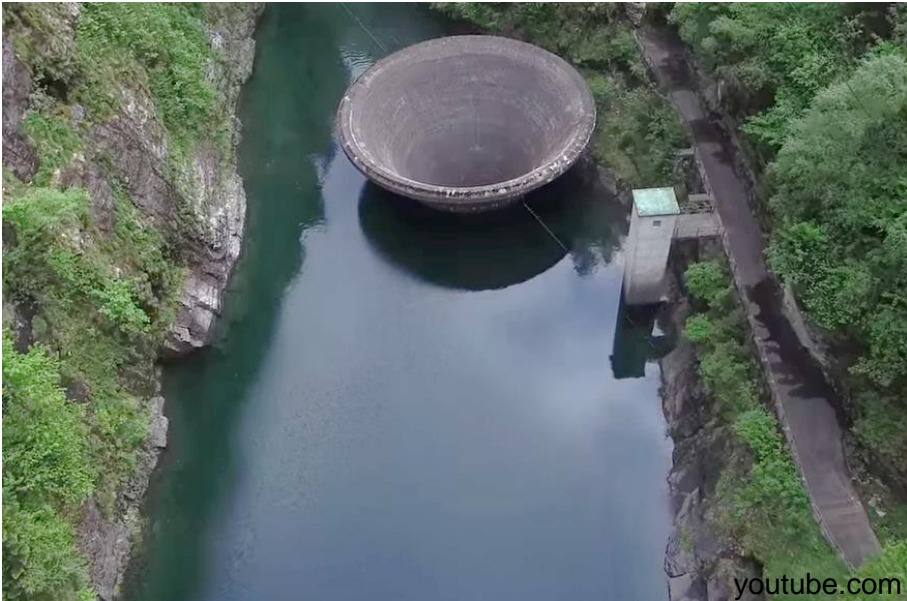
Moring glory (spillway)
