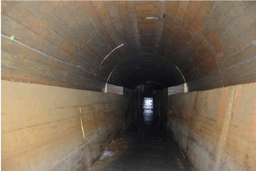
Bottom outlet gate (outlet tunnel)
