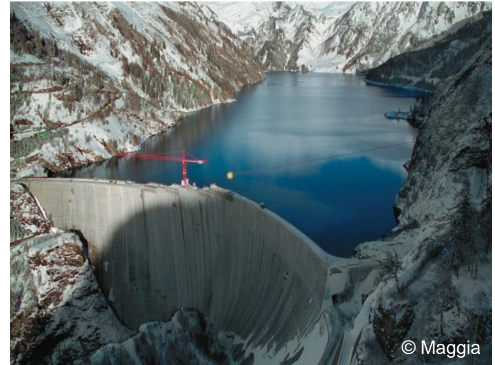
Dam heightening Luzzone (1998)
