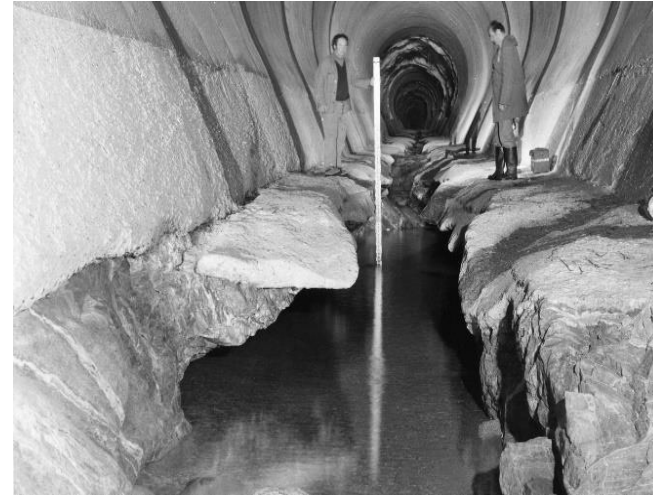
Palagnedra SBT, Switzerland (Photo: VAW, ETHZ)
