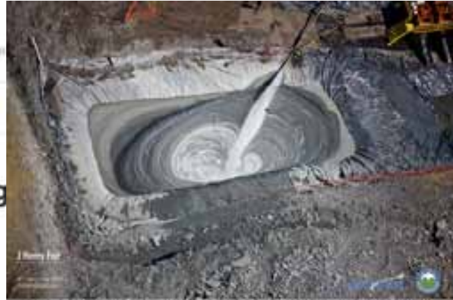
(Drilling fluid splashing past the liner, Dimock, PA, Spring 2009)
