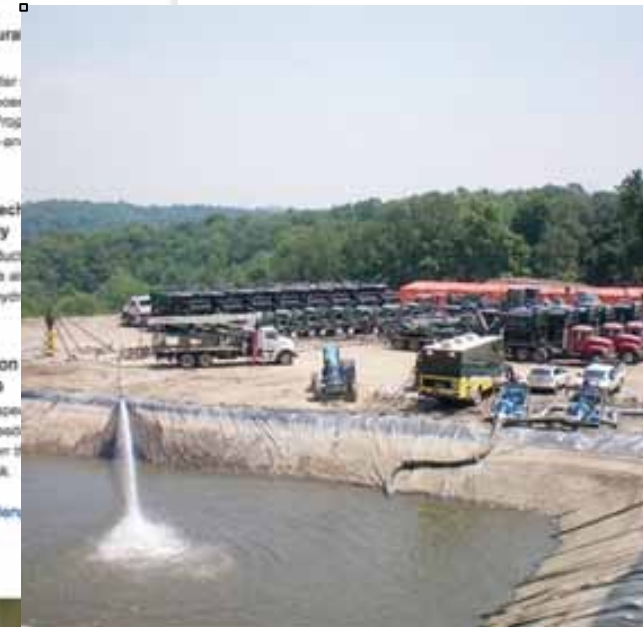
(Drilling fluid splashing past the liner, Dimock, PA, Spring 2009)
