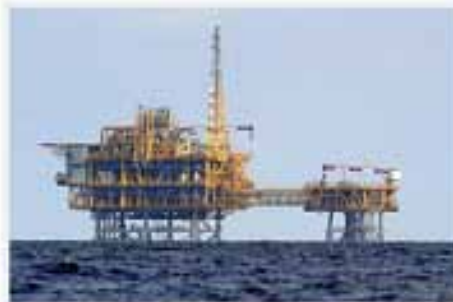
A platform, part of the Castor Project, located in the Ebro Delta off the coast of Alcanar stands at sea on October 2, 2013 following ten earthquakes with a magnitude between 1.4 and 2.9 registered today and
