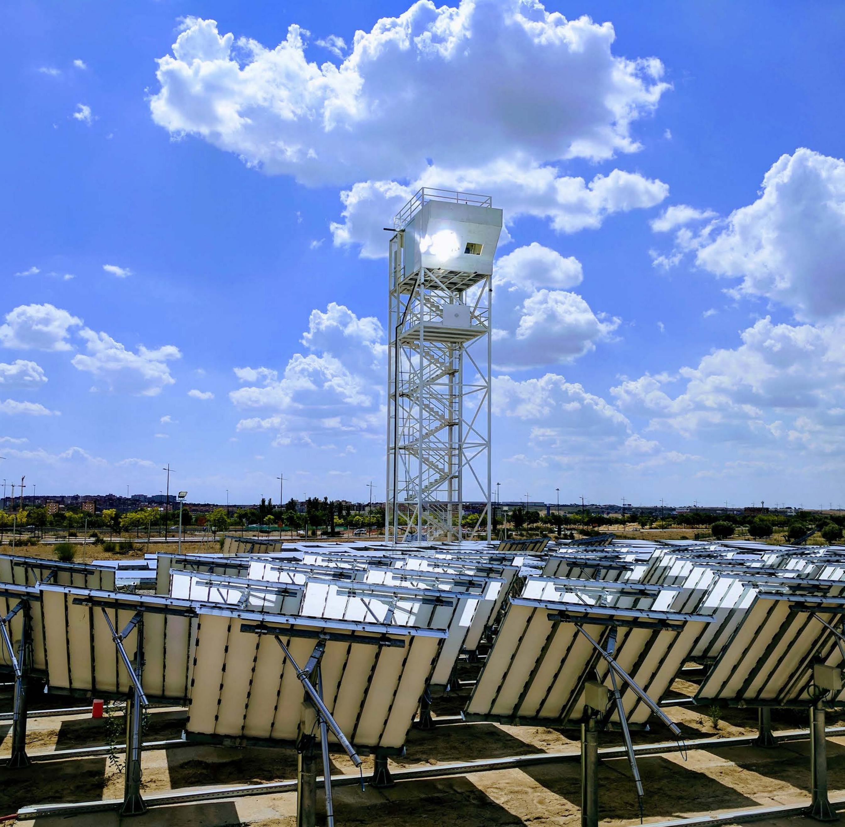
Fig. 3: Photograph of the solar tower fuel plant located at IMDEA-Energy, Madrid. A field of sun-tracking heliostats focuses the direct solar irradiation onto the solar reactor positioned at the top of the tower. The solar reactor co-splits \text{CO}_2 and \text{H}_2\text{O} via the ceria-based thermochemical redox cycle and produces a desired mixture of \text{CO} and \text{H}_2 (syngas), which is finally processed via Fischer-Tropsch synthesis to kerosene [4].
