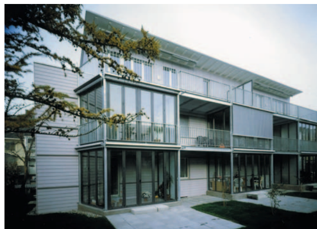
Fig. 4.1-3: Retrofit Demonstration Building Therwil (CH): after renovation and added penthouse, 1/4 of original energy demand for heating and hot water (~ 50 kWh/m 2 )
