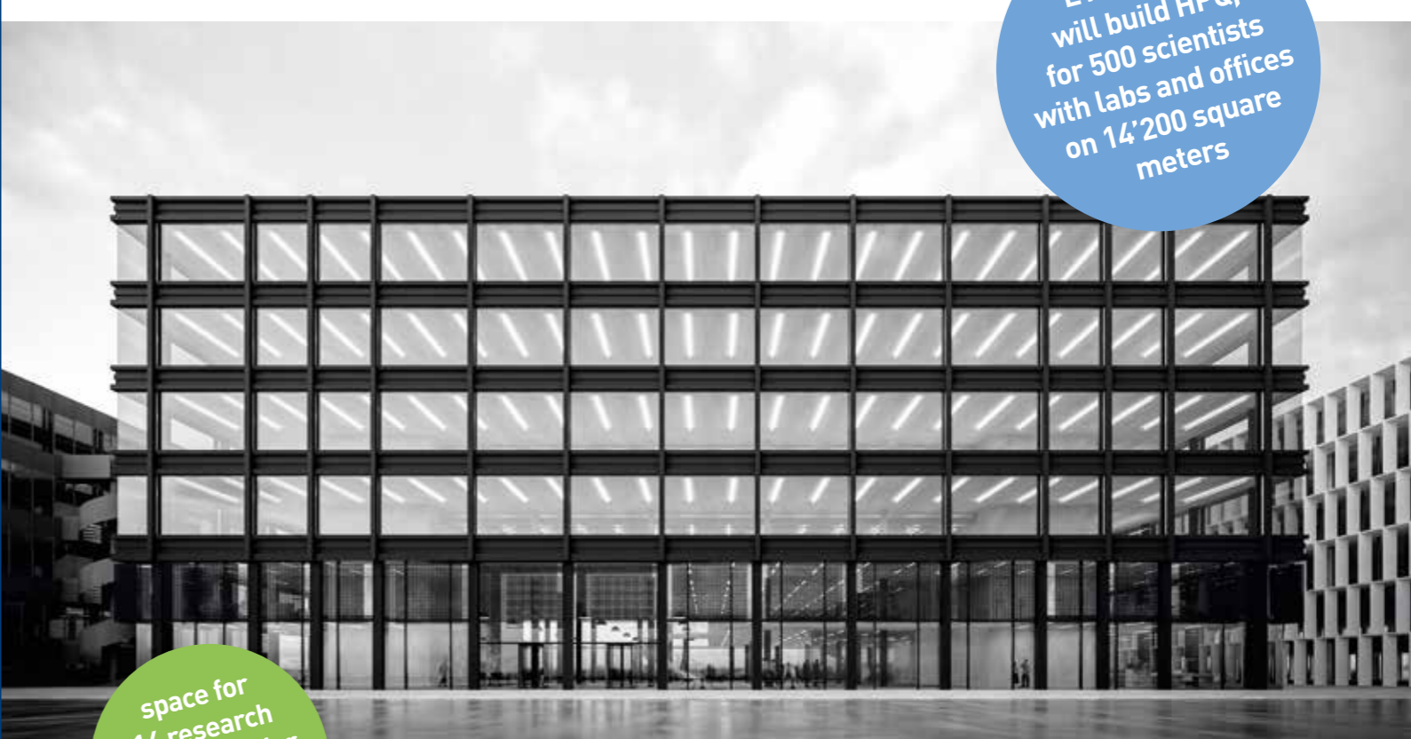
View from the south-east on the façade of the HPQ building at the Wolfgang-Pauli-Strasse (in the front). The HPQ building is embedded between the HIF (left) and HIT (right) buildings. The double height entrance involves a mezzanine (left and right). Additional four floors hold office space (at the periphery) and lab space (in the center of the building).
