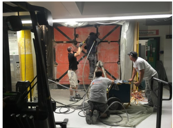
Fig. 3: Dismantling the concrete door with heavy equipment in the control room.
