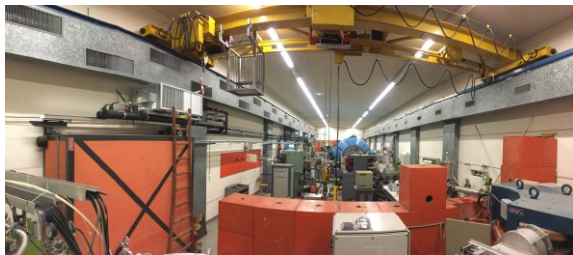
Fig. 1: Removing the concrete shielding blocks in the Tandem hall, the concrete door at the left was also dismantled and removed.
