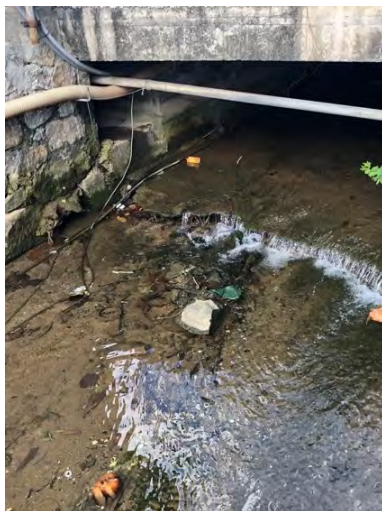
Figure 42: Example of a non-continuous bed substrate beneath a road (Rivière Moussa, own source, 14/03/2019).
