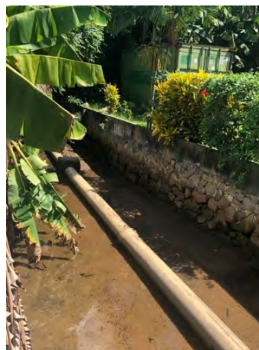
Figure 25: A bank bed in medium condition (English River, own source, 13/04/2019).
