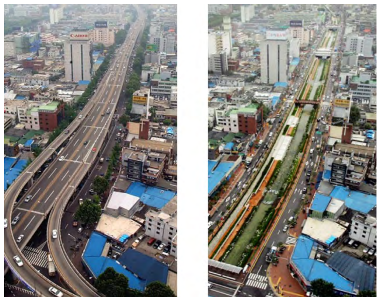
Figure 3: State of the Cheonggyecheon river before (left) and after (right) the restoration project (Woo, 2010).
