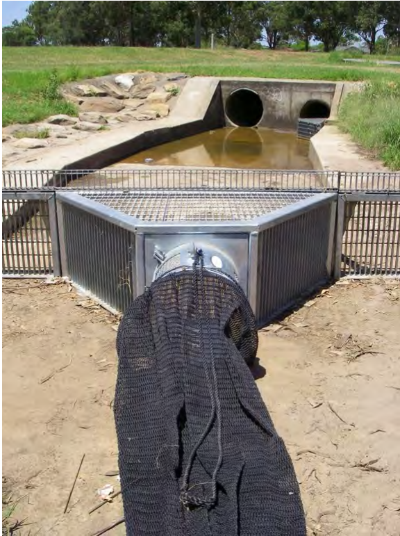
Appendix UU: Example of a trash trap (Storm water systems, 2019).
