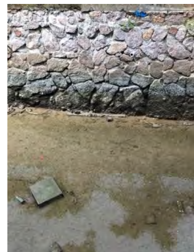
Figure 26: An impermeable bank bed in a good condition (English River, own source, 18/04/2019).
