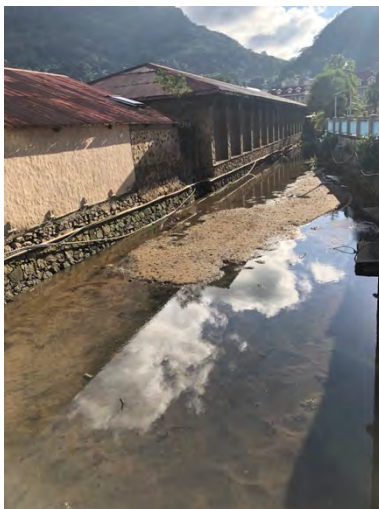
Figure 29: Further channel structure (gravel accumulation) in Rivière Moussa (own source, 27/03/2019).
