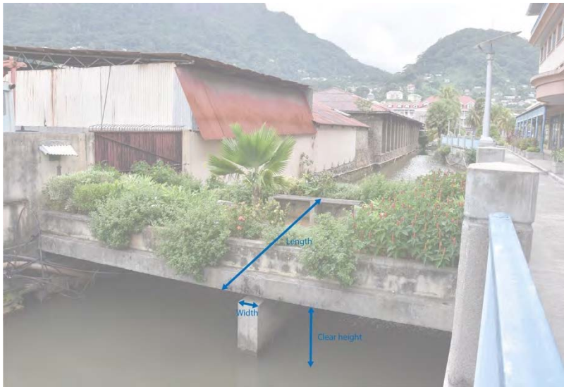
Figure 41: Small picnic area above the river illustrating the clear height, width and length of an object (Rivière Moussa, own source, 10/03/2019).
