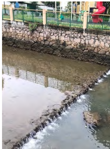
Figure 19: Example of large construction of bed with impermeable material (Rivière Moussa, own source, 14/04/2019).
