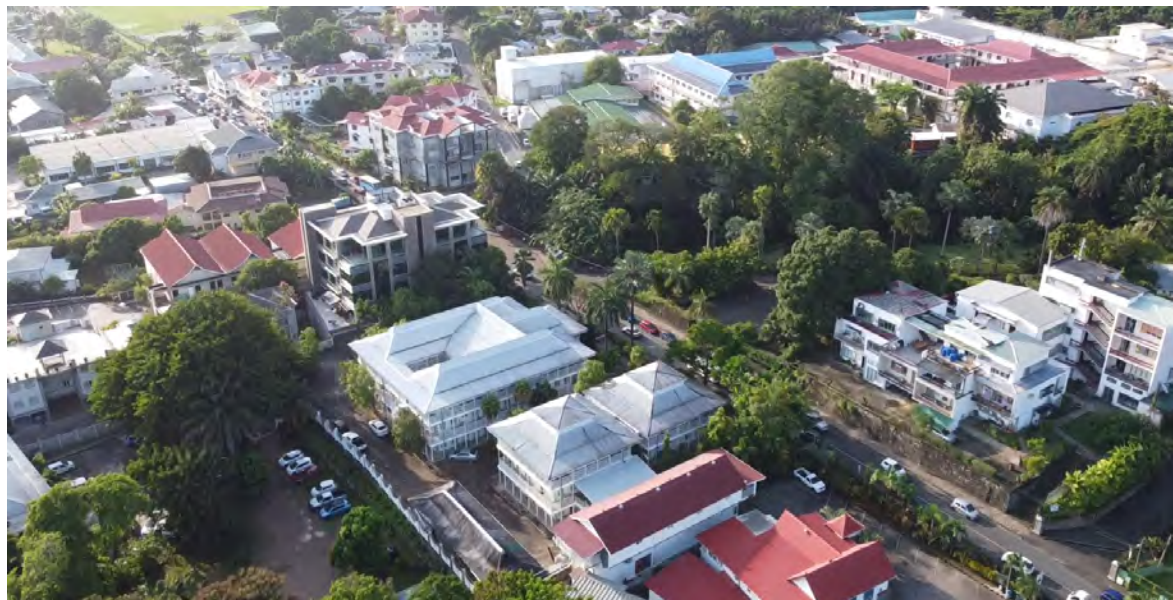
Figure 3.13: Example from congestion checks with drone imagery at Mont Flery Road (February 2022).
